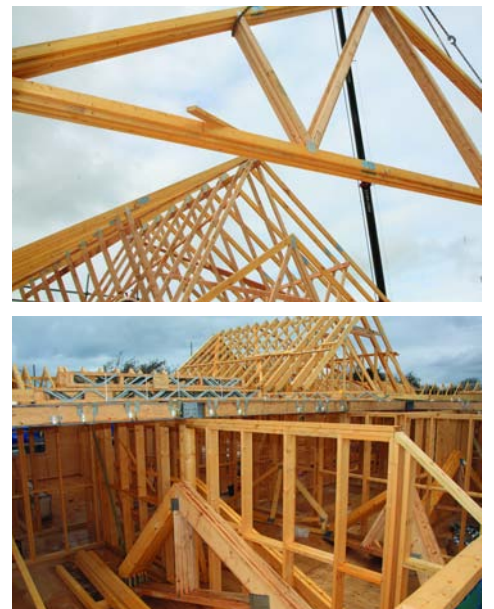
Engineered roof trusses.
